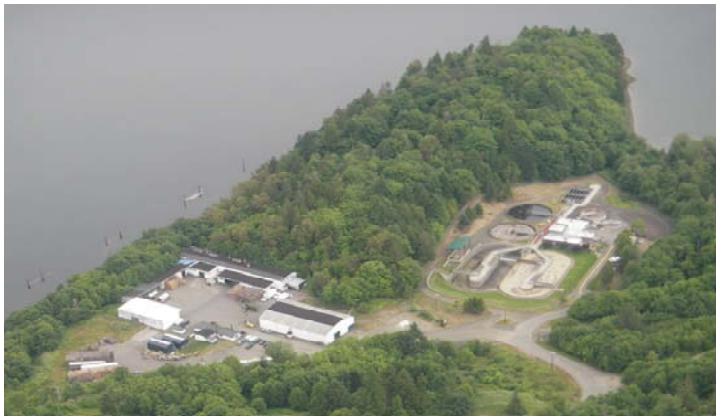
The Shelton Wastewater Treatment Plant site, as it looks today.
